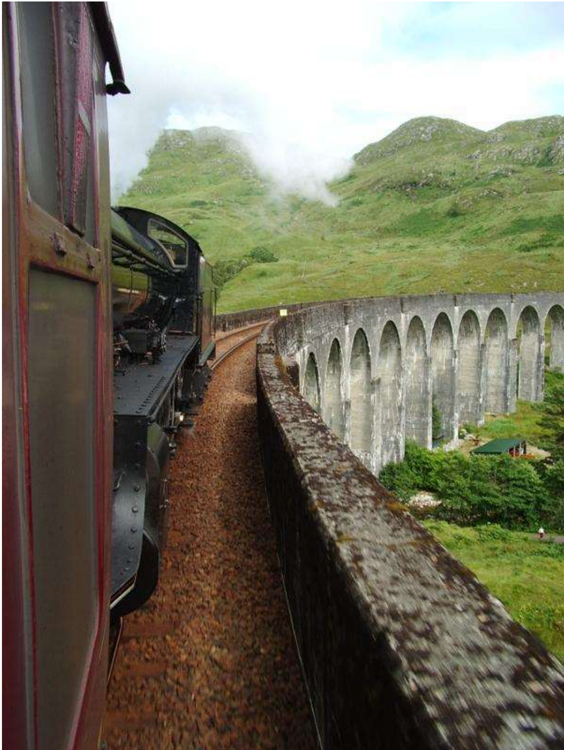
Leaving Glenfinnan on the way back to Fort William, the train crosses the Glenfinnan Viaduct, now famous as the 'Harry Potter' viaduct.
