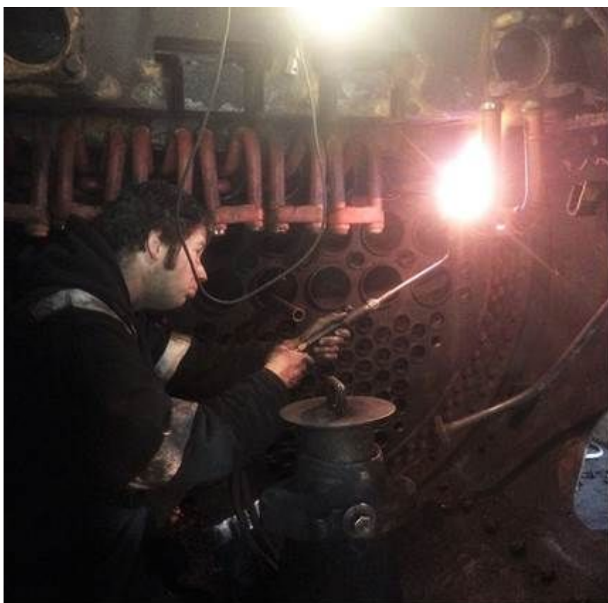
Chris heats up elements ready for bending to fit. Photo courtesy of Dave Fowler.
